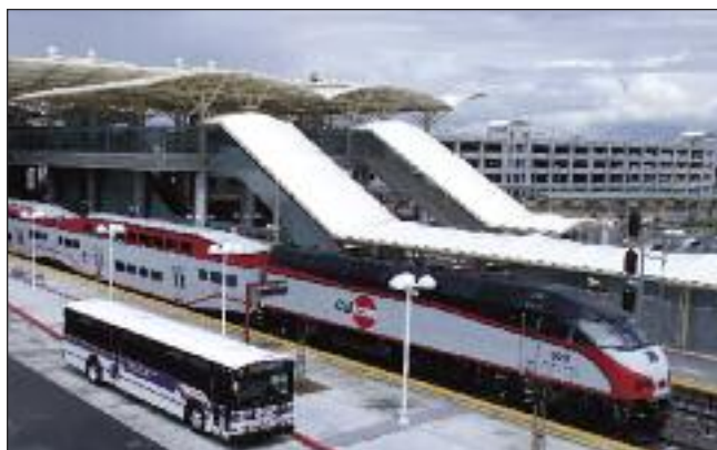
The existing multimodal BART/Caltrain station in Millbrae
